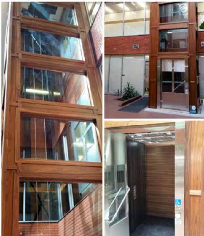
Figure 1: A full-height-carriage lift; photos courtesy of Uppercut Elevators and Lifts
